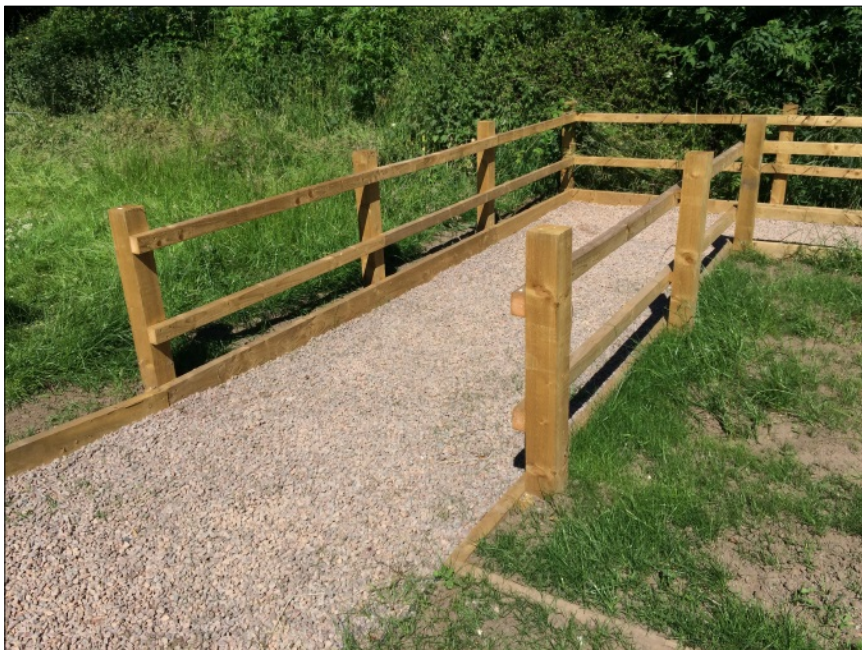
Photograph of new footpath.
